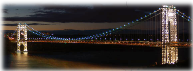
George Washington Bridge
